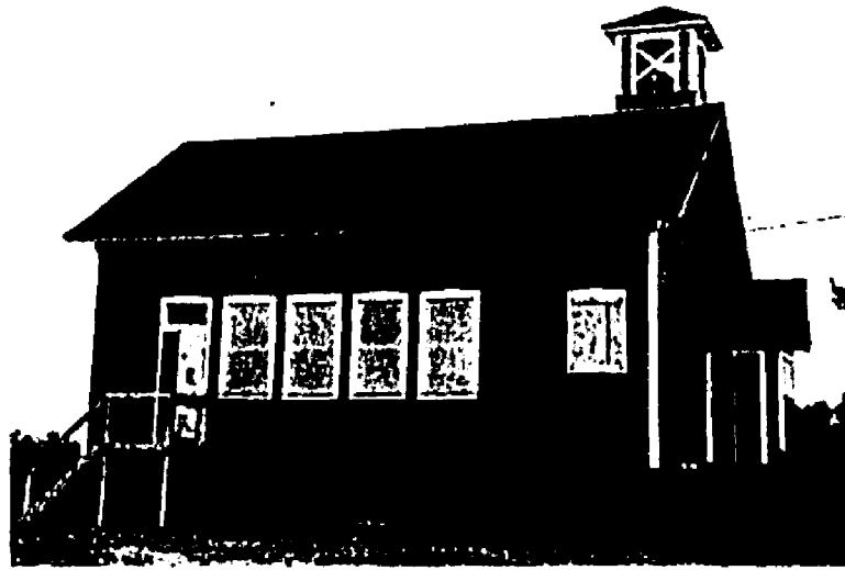
Figure 103. Schoolhouse with Protective Fiberglass Shutters in Place
