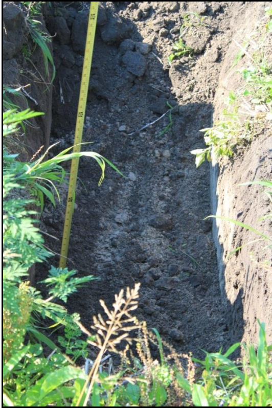
Figure 2. Hole dug by backhoe with proper length, width, and depth measured.
