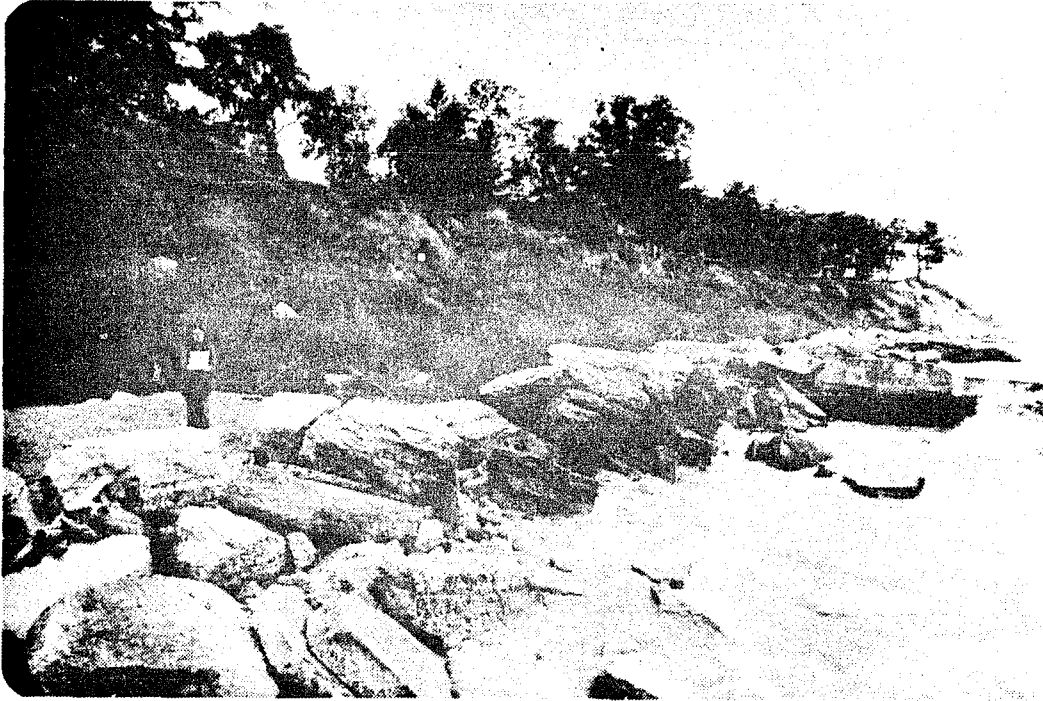
Figure 29. Bluff protection measures in the North \frac{1}{2} / Section 8 / T2N,R23E, Kenosha County, Wisconsin. This photo was taken on July 30, 1978
