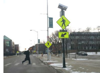
Rectangular Rapid Flashing Beacon
