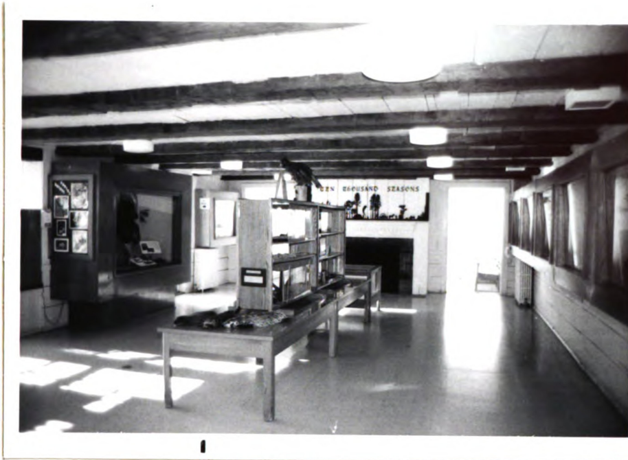
Figure 2. Exhibit Room, Stony Creek Nature Center, West
