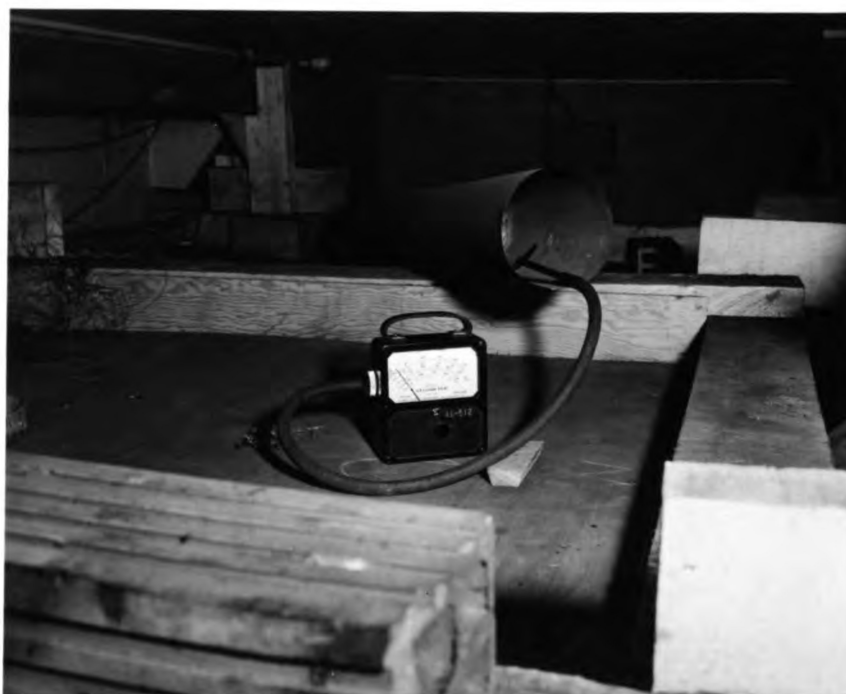
Fig. 10 Measuring the Air Flow.
