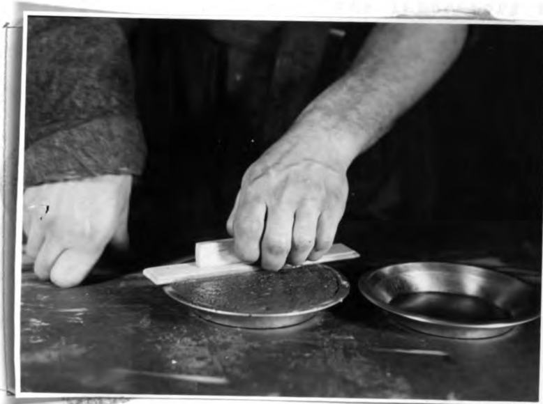
FINISHING WITH WOOD FLOAT
