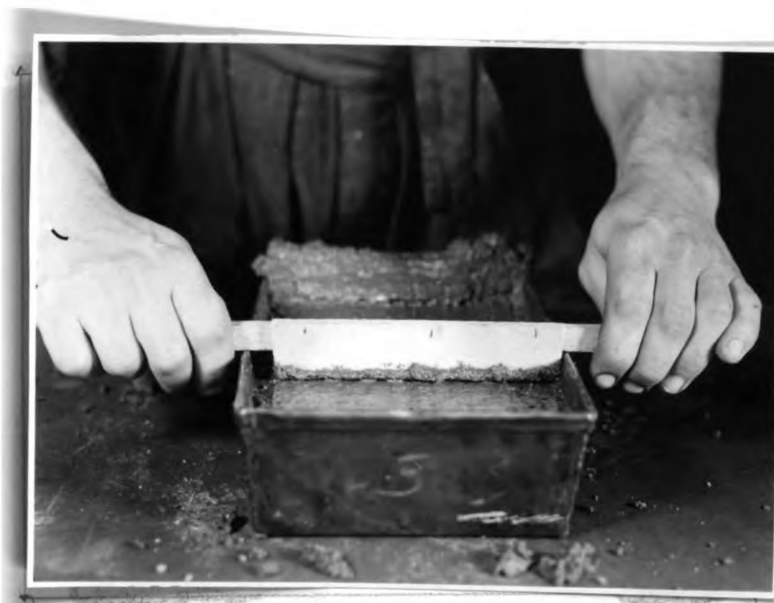
FINISHING WITH STRIKE-OFF
