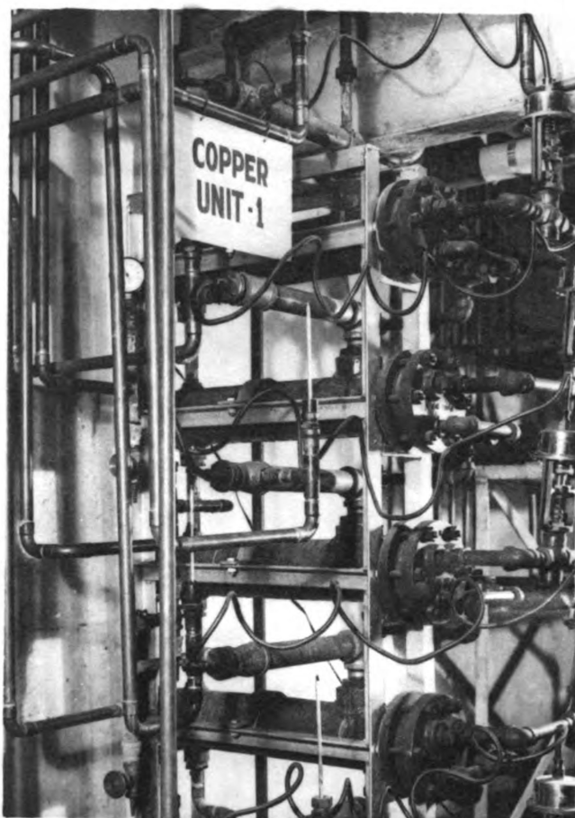
Figure 4. Test Panel Heat Exchangers
