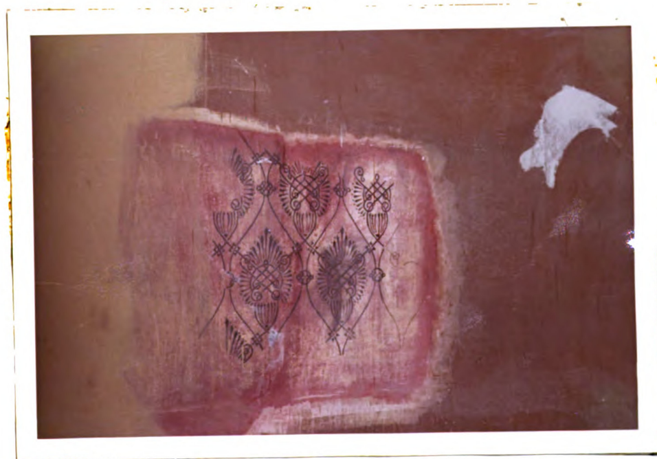
Fig. 27.—An example of the recast plaster pieces used in the restoration.
