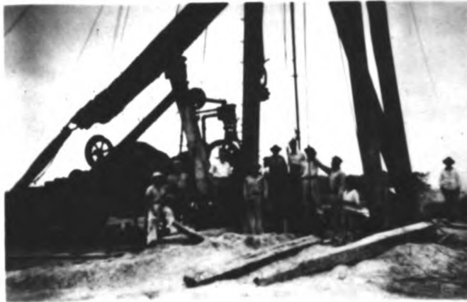
Plate 2.- A cable tool for shallow wells Commonly used in Cautivo (La Libertad).
