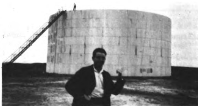
Plate 5.- Tank for crude oil (50,000 bbl.) La Libertad, Ecuador. Oil tank is without sand fire wall to prevent loss of oil or spread of fire in case of accidental break.
