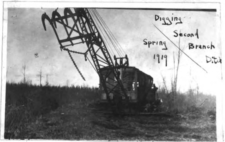
"Walking" Gasoline Dredge Using Brush Hooks. (1919)
