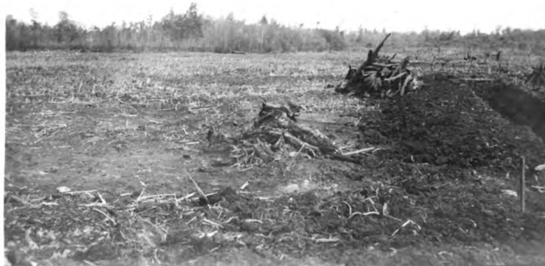
Beginning Hand Ditch
