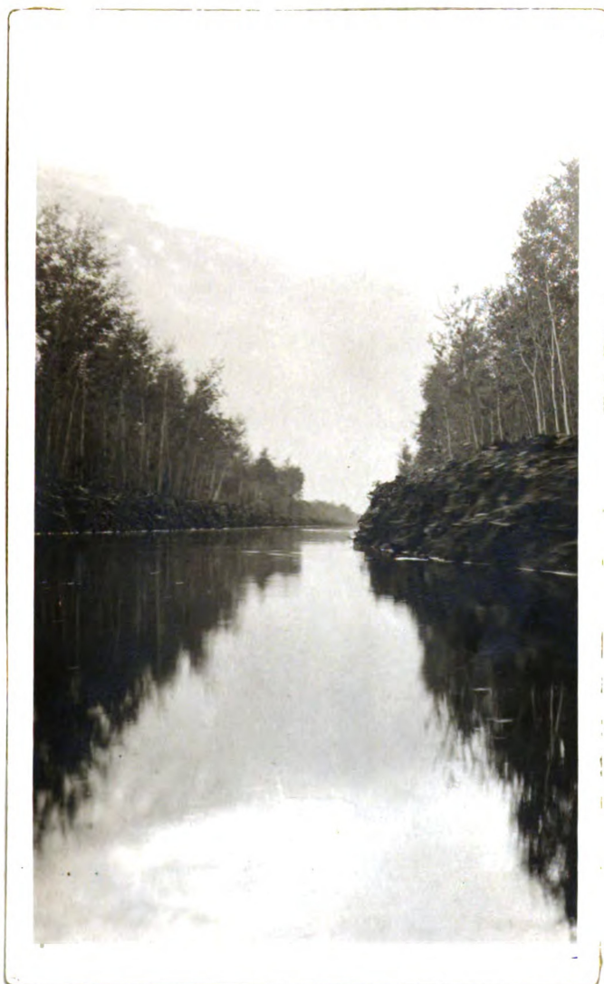
Beaver Drain, before Completion of Outlet
