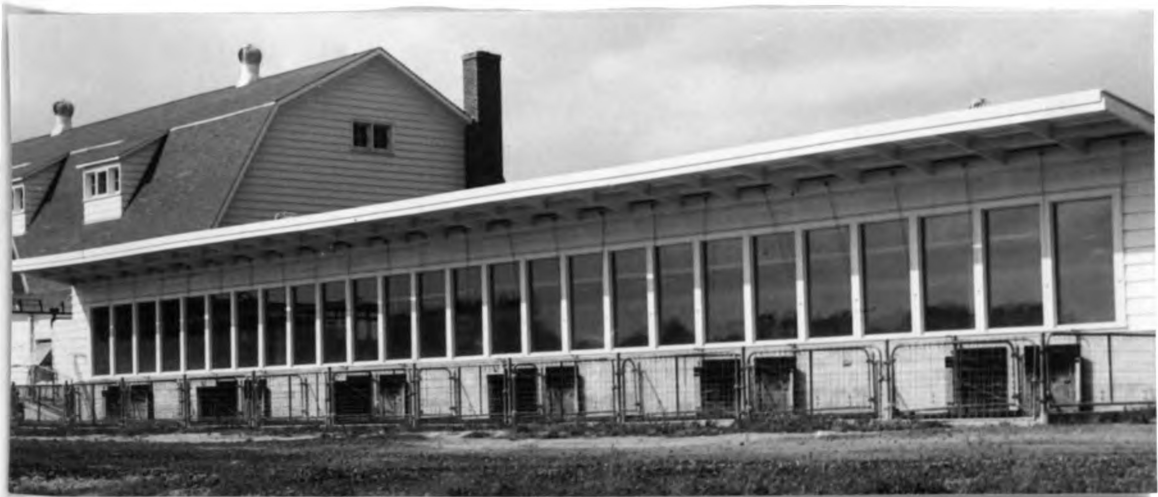
Fig. 3. Exterior view of solar wing on September 22, 1952; overhang in "extended" position.
