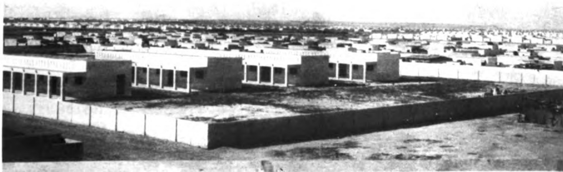
One of the eleven primary schools provided in the Korangi Township
