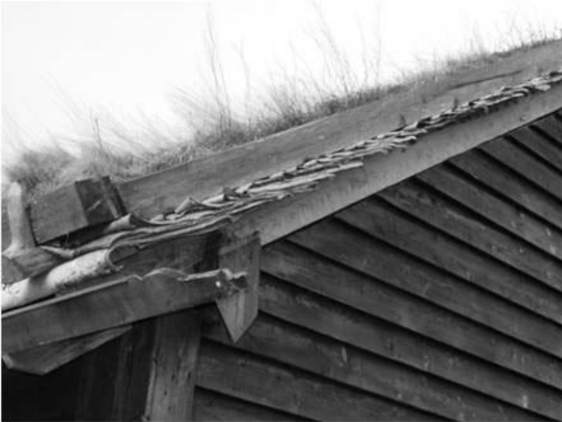
Example of early birch bark waterproof membrane technique. Scandinavian cabin, West Norwegian Folk-Art Institute, Voss, Norway (Photo courtesy of Westphal 2008).
