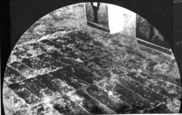
Above—Single Tamping Block Weighing 2\frac{1}{2} Tons. At Right—Multiple Tamping Machine. Below—Close-up of Consolidation Obtained by the Use of Tamping Equipment.
