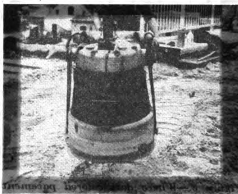
Figure 12G "Jumping Frog" used to compact cohesionless sand.
