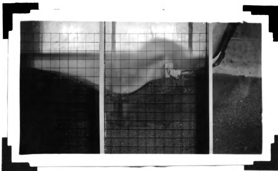
This shows the erosion during a large head with the stilling dam four inches from the toe of the dam.
