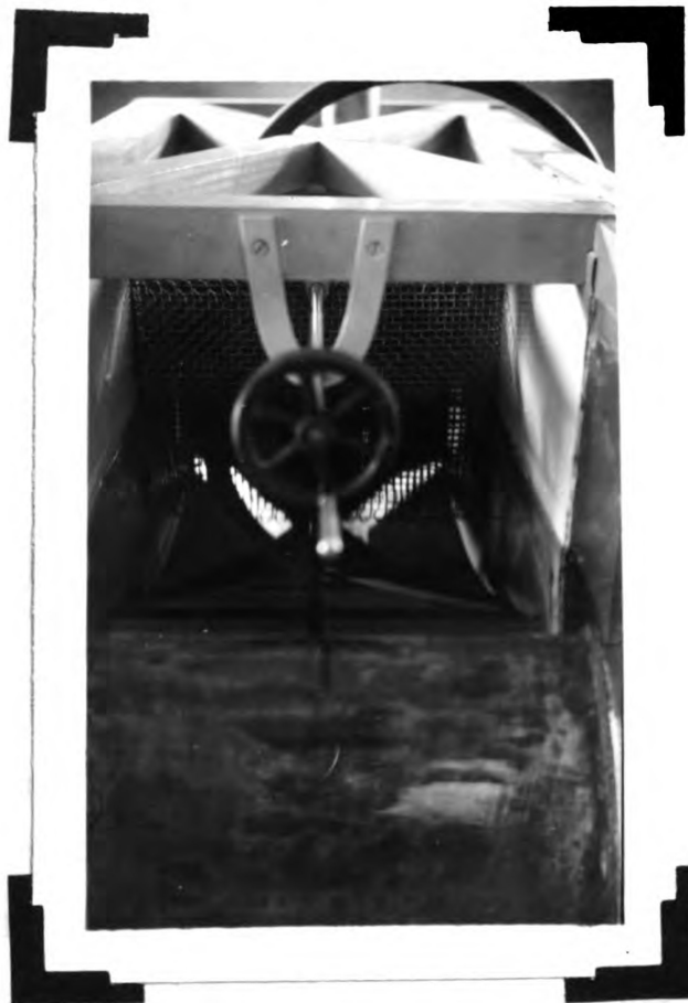
View over top of dam showing the hand wheel and the second screen baffle. Notice the stillness of the water going over the dam.
