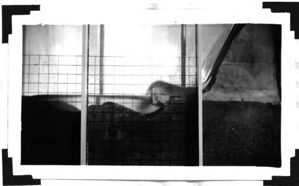
This shows the shape of the erosion when a large flow is followed by a small flow, stilling dam four inches from the edge of the toe. Note how the erosion goes back under the apron.
