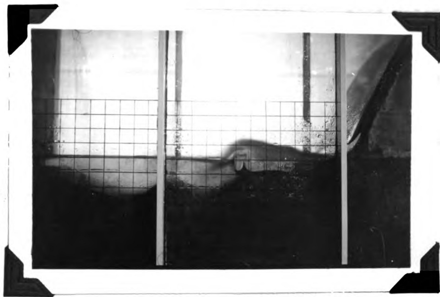
Effect of a small flow following a large flow, note how the erosion has moved toward the stilling dam
