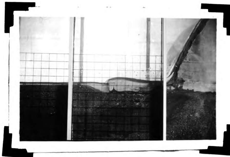
Stilling dam six inches from the toe with a small head and low tail-water
