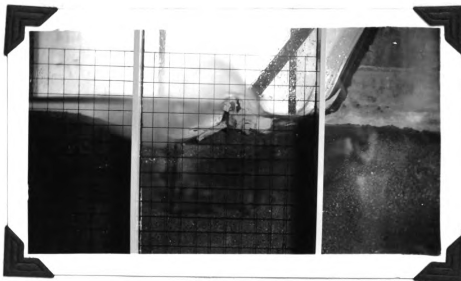
This shows the same stilling dam during a large flow. Note how the water shoots into the air after leaving the stilling dam.
