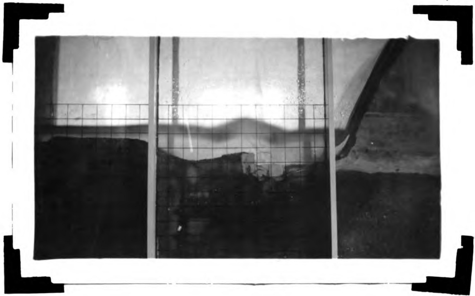
This shows the stilling dam five inches from the toe with a small flow and high tail-water
