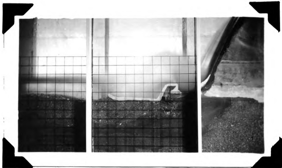
Stilling dam and pool same as above during a large flow with ordinary depth of tail-water
