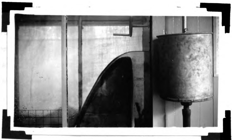
Side view showing the water going over the dam. The hook gauge and tank are at the right.
