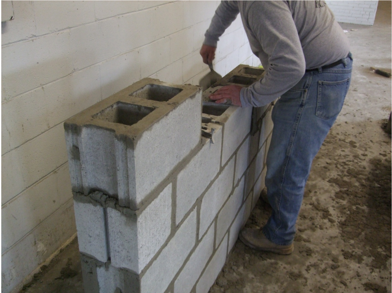
Figure E.6: Constructing with traditional masonry units.
