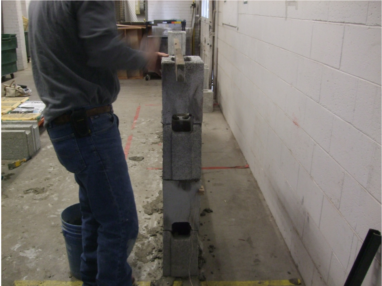
Figure E.5: Constructing with refined masonry system.
