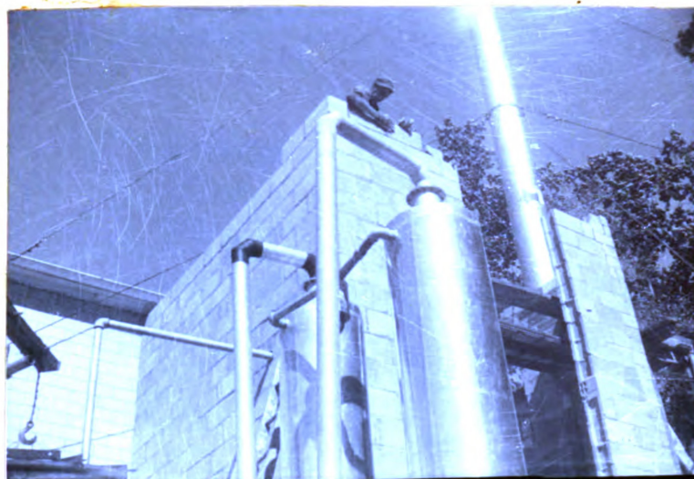
Figure 25. The blackened portions on the four-inch aluminum pipe locate the vapor leaks before repairs. The wall housing the boiler is nearing completion. The pipe was dismantled welded and then replaced to stop the leaks.
