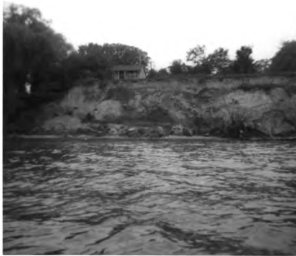
Fig. 1- Eroded cliff, southern end of Lexington village limits
