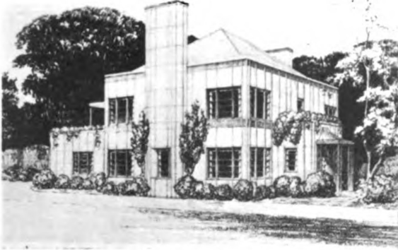
FIRST PORCELAIN-ENAMEL HOUSE , sponsored by the Ferro Enamel Corporation is under construction in Cleveland. Exterior porcelain-enamel sheets are \frac{1}{2} " deep, panels varying in size up to about 30" square and "sandwiching" a fiber insulating board held by a waterproof glue. Special steel studs are fabricated. Horizontal joints have a slight ship-lap. The total wall thickness is about 4 inches. Charles Bacon Rowley and Associates are the architects and engineers, with Meade Ashley Spencer as associate.
