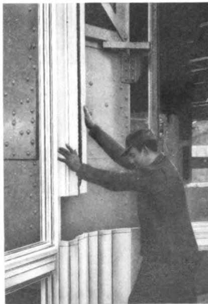
Extruded aluminum window and pier construction and erection method—also the expansion joint provided at each floor.
