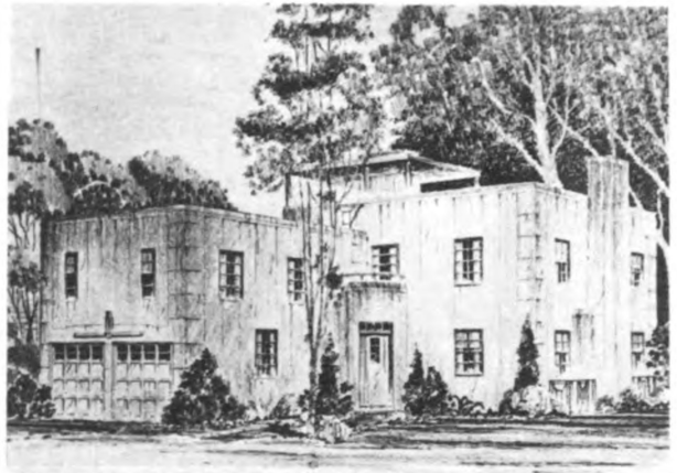
EXPERIMENTAL FRAMELESS STEEL HOUSE erected in a Cleveland suburb by the Insulated Steel Floor and Wall Company. Stamped steel sheets are used for the construction of floors and walls. Overlapping joints are welded and a filling of mineral wool is used for insulation between the steel sheets. This system of construction is said to have unusual heat and sound insulating qualities, and a flexibility which makes it adaptable to almost any type of building. The experimental work is under the direction of Mills G. Clark of the American Rolling Mill Company.
