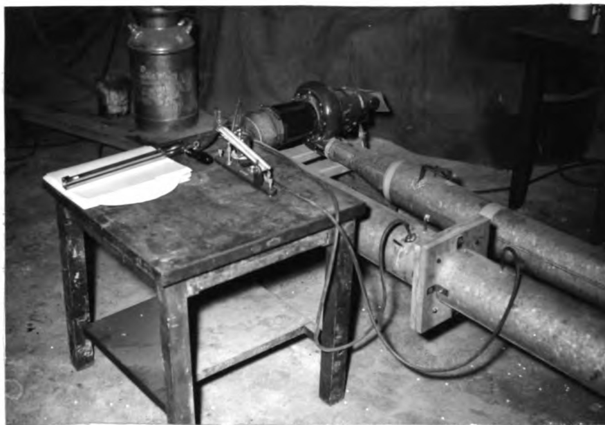
Fig. 11. Measuring Air Flow in Return Duct
