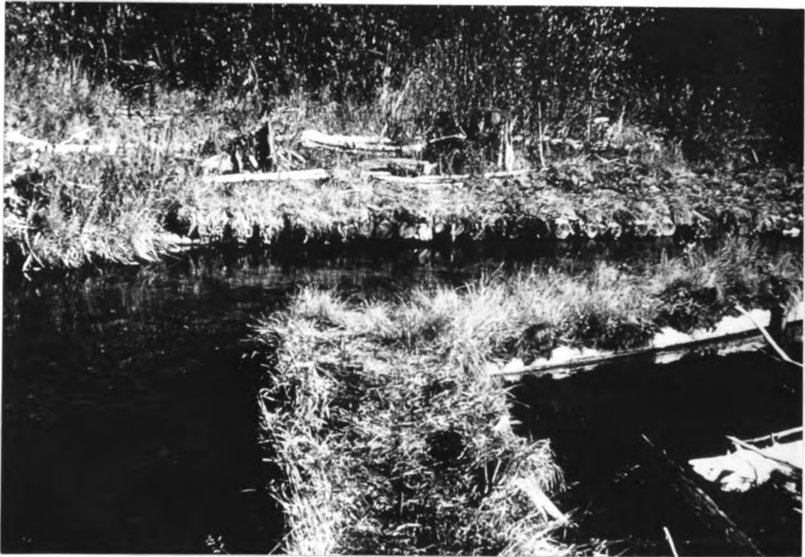
Figure 24. Single-wing deflector (crib-type) with log-sog cover on opposite bank--Evergreen River.
