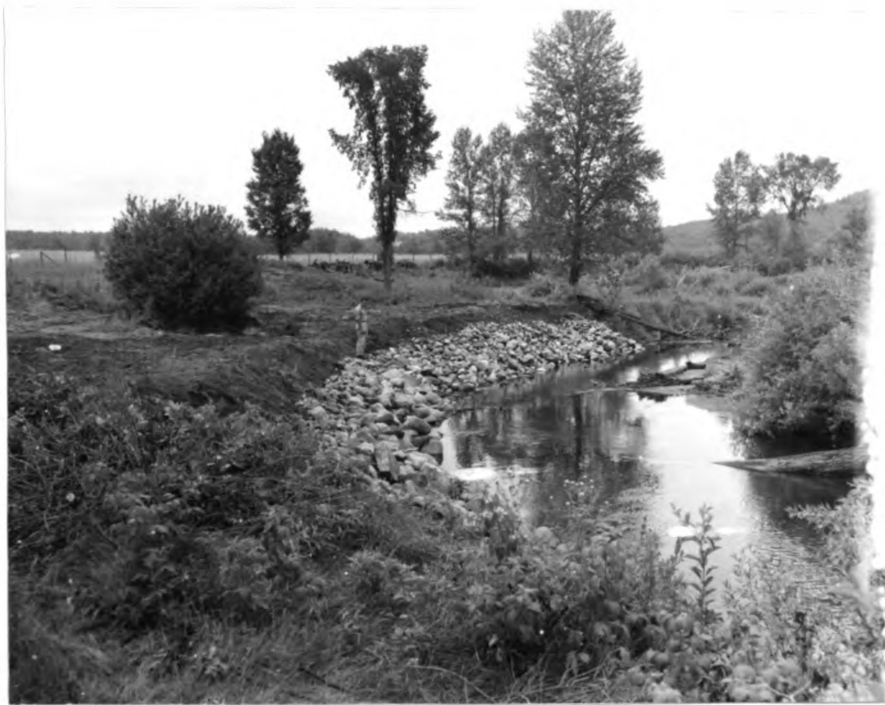
Figure 19. Same streambank after bank stabilization with rock riprap. (Michigan Department of Conservation, LSI, Photo.)
