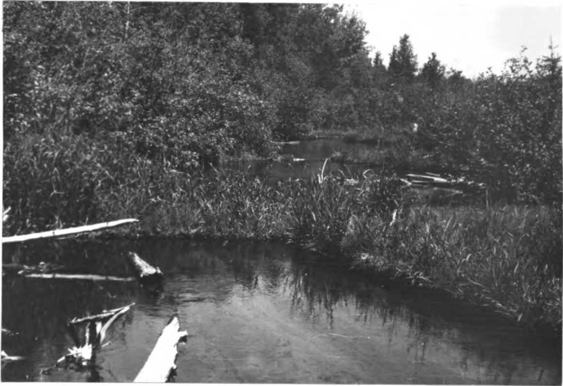
Figure 25. Digger logs with log sod cover--Evergreen River Cooperative Stream Improvement Project.
