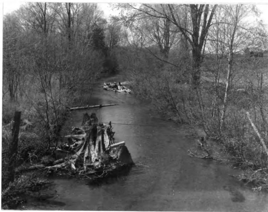
Figure 14. In-stream devices--stump cover (lower left), log cover (downstream on right). Cedar River, Gladwin County, Michigan. (Michigan Department of Conservation, LSI, Photo.)
