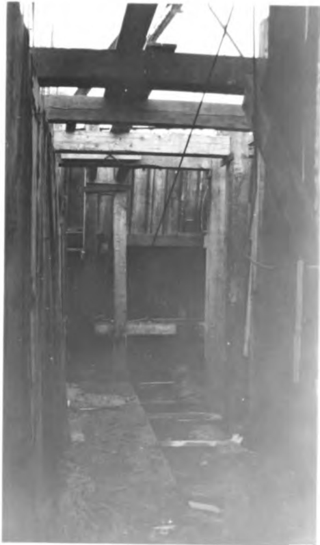
New method of bracing with vertical posts and overhead struts. Note bracing against footing.
