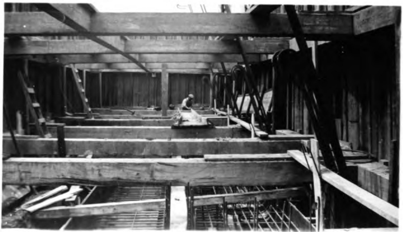
Struts and walers plus some rein- forcing steel.
