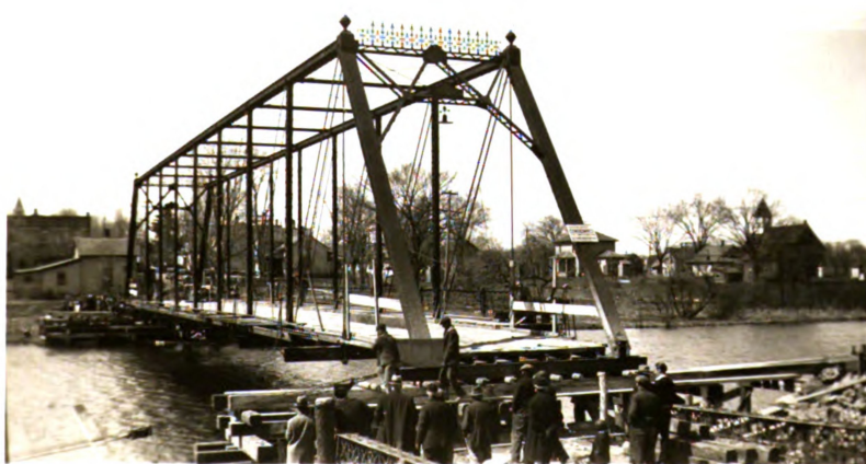
Bridge being moved. Note timber cribbing at left.
