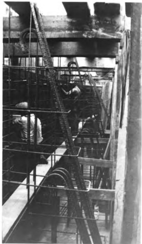
Reinforcing steel. Large rods at an angle are for counterforts.
