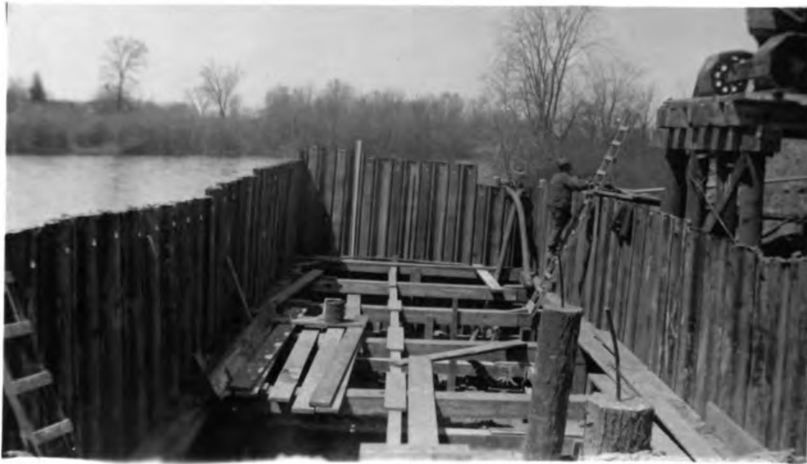
Regular method of bracing.
