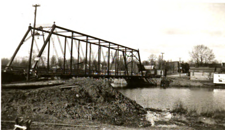
The old bridge, built in 1894, showing old position, with fill for new (temporary) roadway in place.
