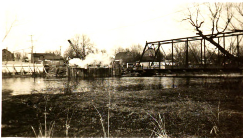
Driving sheet-piling
