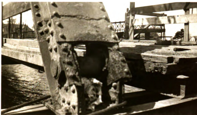
The necessity for a new bridge, showing rusted and cracked members on the old truss bridge.
