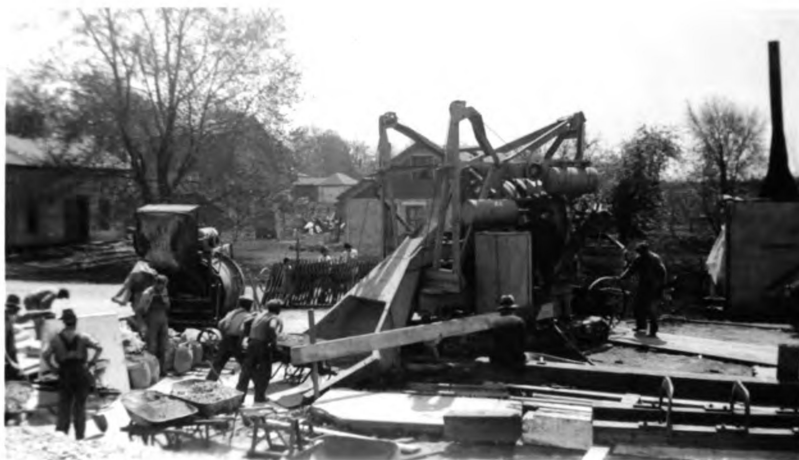
Detail of pouring layout. Note extra mixer for breakdowns.
