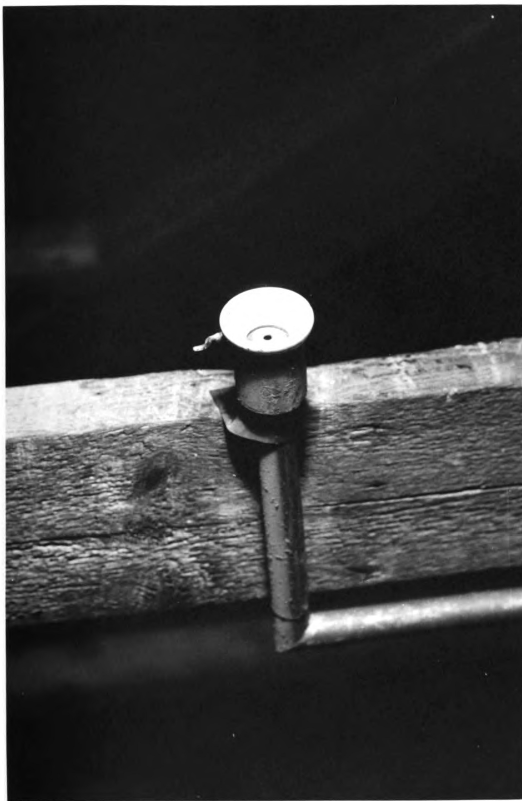
Fig. 12. Voice Tube from Fly Gallery to Stage.
