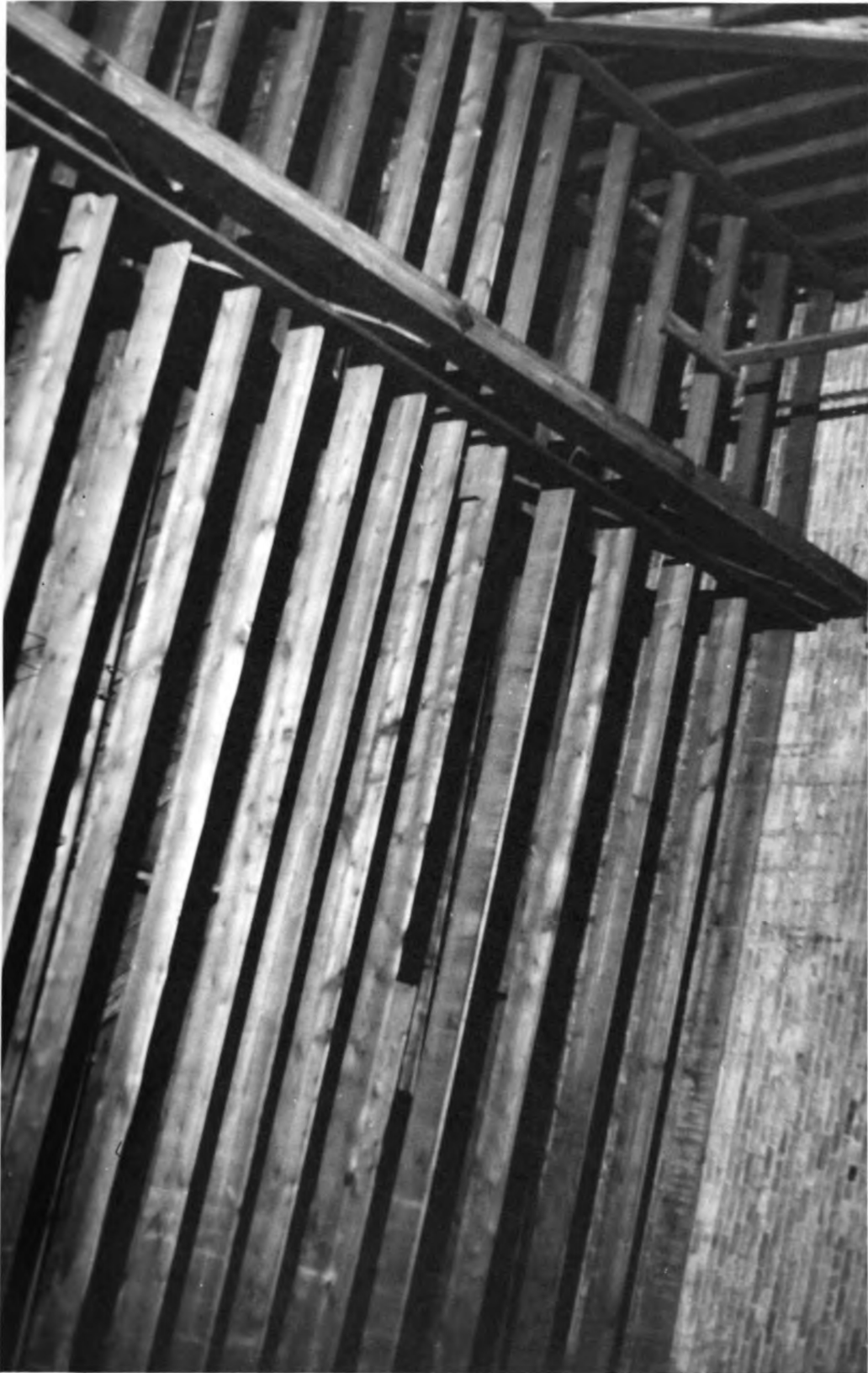
Fig. 11. Gridiron showing Support Truss. Note that the grid supports run up and down stage.
