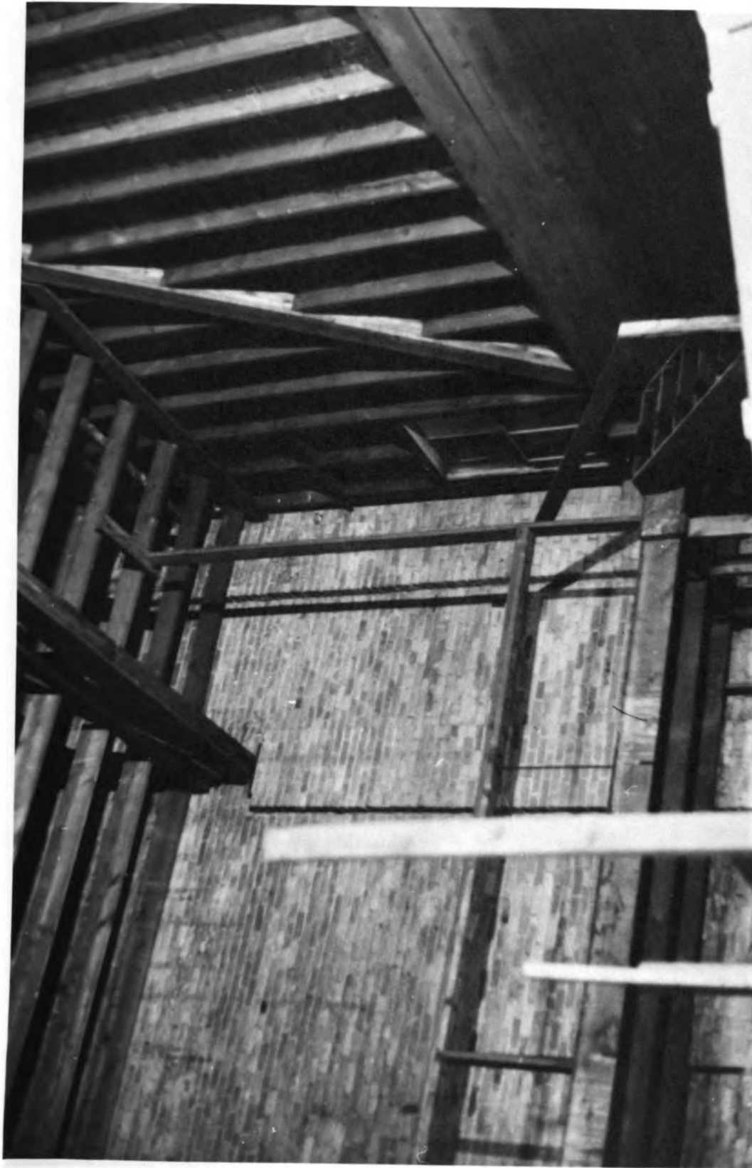
Fig. 10. SL Fly Gallery. Note truss support at center and proscenium wall at the right.
