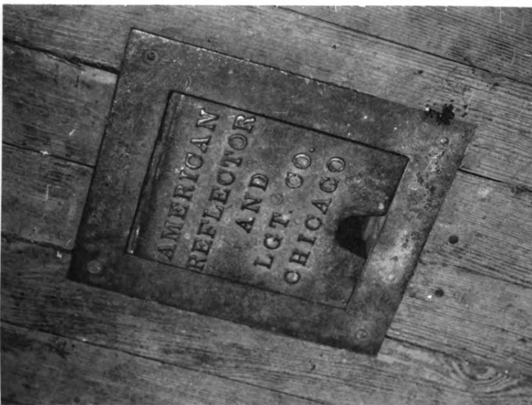
Fig. 6. SR Electric Floor Pocket.
