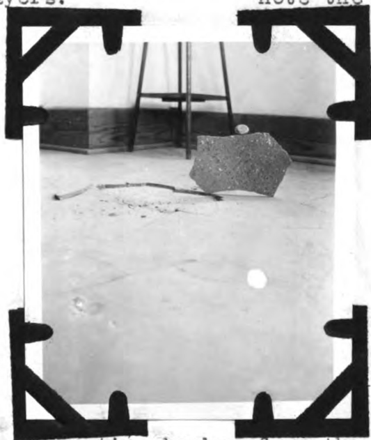
a section broken from the floor noted in the first part of this discussion.
