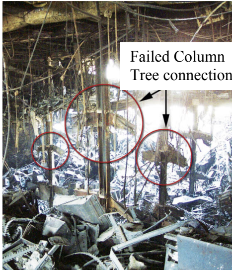
(c) Failed column tree connections and after fire structural damage
