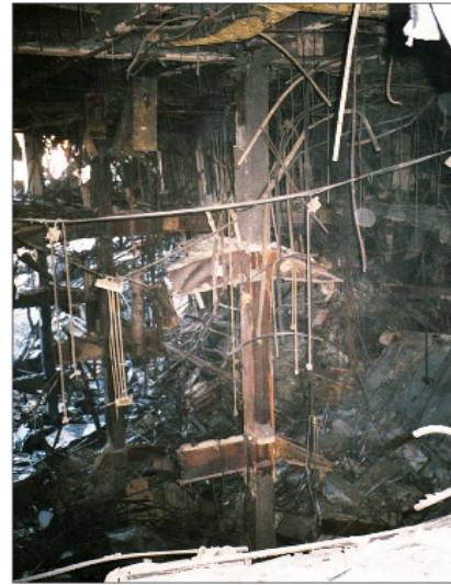
(d) Failed column tree connection and floor assembly without significant damage to column
