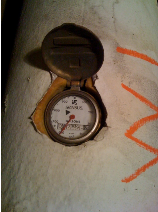
Figure 2: Water Meter (Common Unit) (From MSU Power Plant employee – Rick Johnson, personal communication. 4/29/2010)
