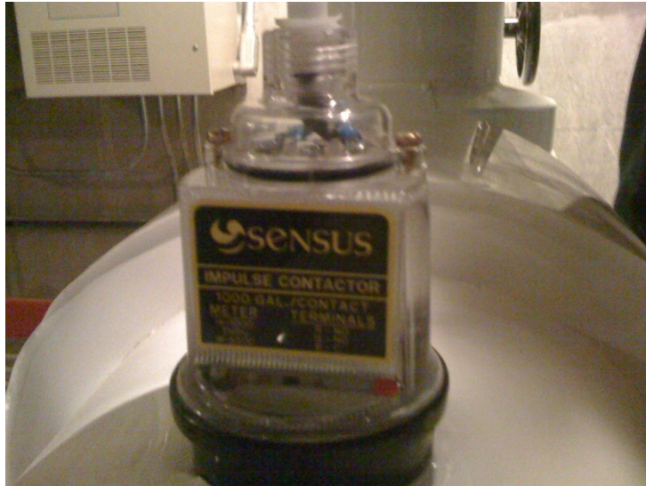
Figure 4: Water Meter (Impulse Unit) (From MSU Power Plant employee – Rick Johnson, personal communication. 4/29/2010)
