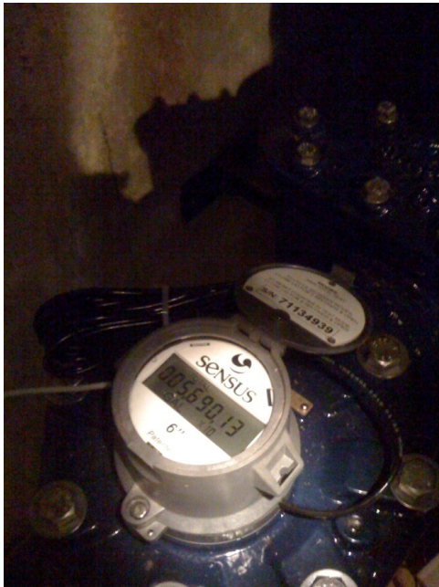
Figure 3: Water Meter (New Unit) (From MSU Power Plant employee – Rick Johnson, personal communication. 4/29/2010)
