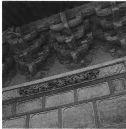
Figure 4-19: Dou-Gong . Chunyang (Pure Positive) Hall, Yongle (Everlasting Happiness) Palace, Ruicheng City, Shanxi Province, Yuan Dynasty (1212 A.D.). Source: Liu, Chinese Architecture (London: Rizzoli International Publications, Inc., 1989), p 133.
