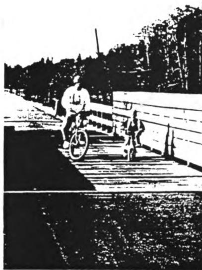
Completed rail-trail bridge
