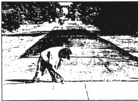
Dewey C. Loper, 46, of RCL Construction in Sanford trowels a concrete approach to the Pere Marquette Rail-Trail at Cedar Street in Sanford.
