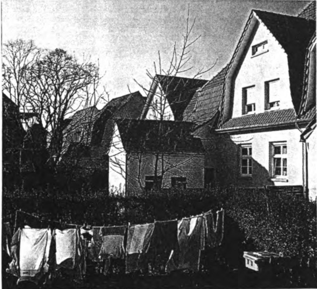
Figure 13. A workers' settlement in Bottrop, one of the largest and most attractive in the Ruhr.
