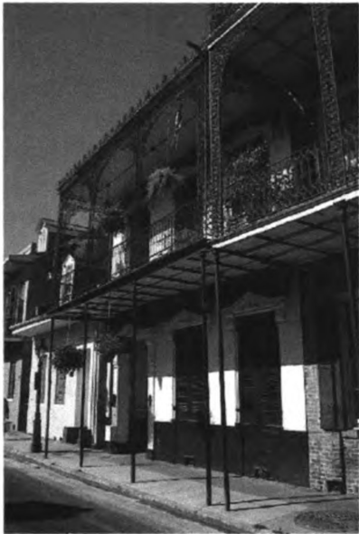
Figure 6. Example of Creole architecture featuring the ubiquitous Vieux Carre balcony and ironwork ( http://www.laimages.com ).
