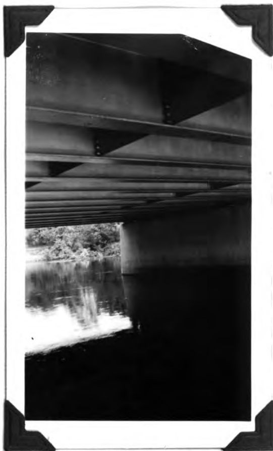
Girders and Piers Showing Intermediate Diaphragms
