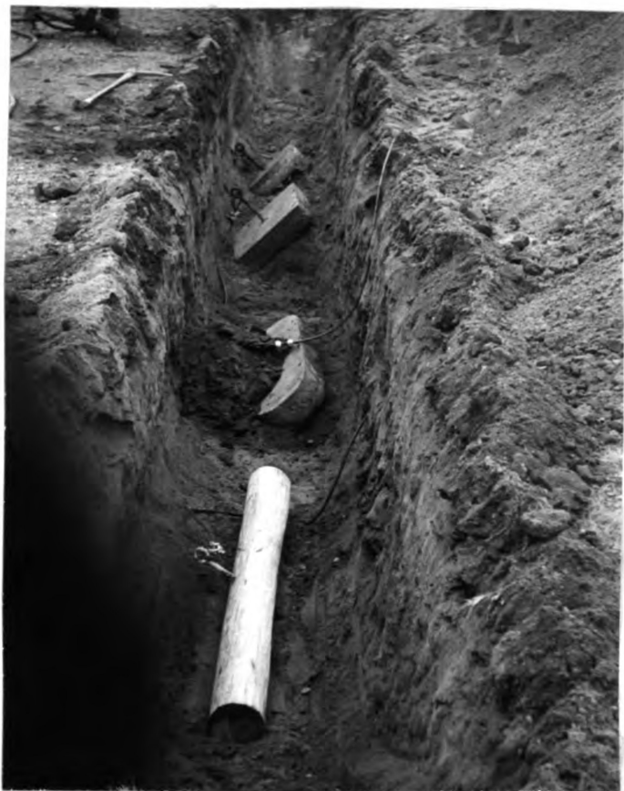
Figure 7. Anchors as placed in the trench.
