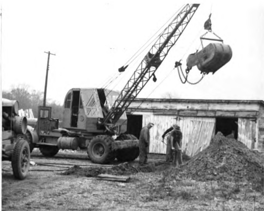
Figure 8. Trench digging and tamping apparatus.
