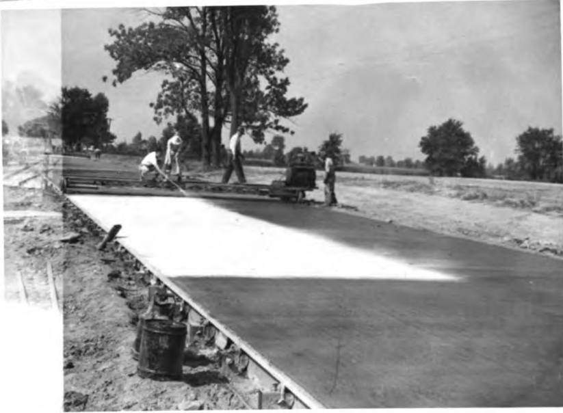
21. Photo indicates initial difference in appearance of white and clear membrane applications (9-17-46). Current spraying equipment for applying clear membrane compounds is shown in background.
