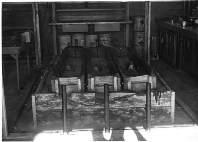
5. Photograph showing beam molds, thermocouple and moisture cells, measuring studs and reference monuments for length change measurements on dry sand subgrade.
