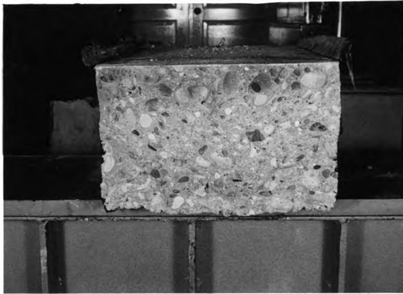
15. Section of beam cured with clear membrane covered with dry burlap-wet sand subgrade. Dehydration line is thin, irregular and not clearly defined.
