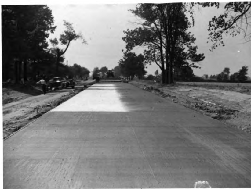
22. General view of pavement after application of membrane films. (9-17-46).
