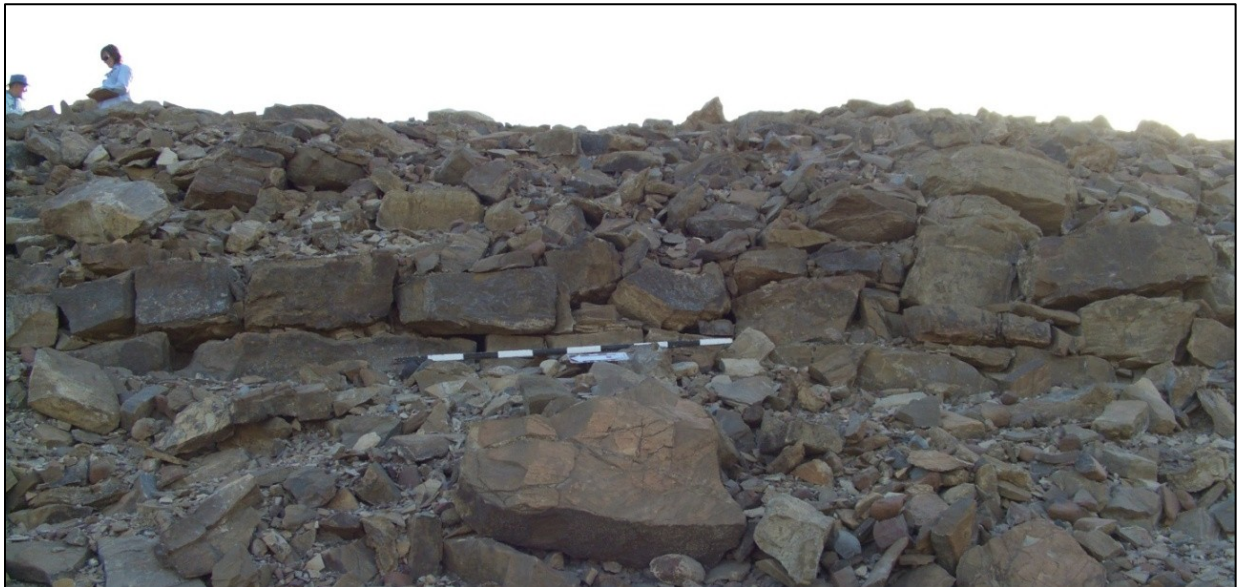
Figure 55. Feature 110980, stone revetment wall downslope.
