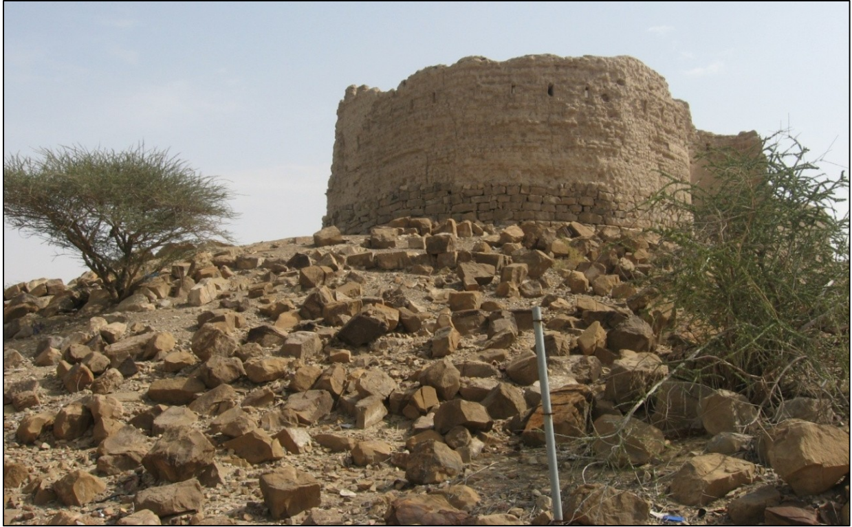
Figure 58. Stone foundation of Wahrah Qala, with rockfall extending downslope. Courtesy of the Bat Archaeological Project
