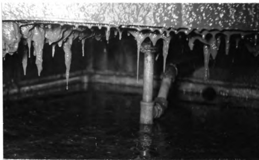
Figure 19. The Under Side of the Filter at the Hydraulic Load of 30.8 mgad.
