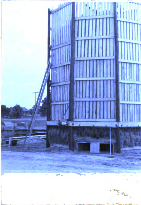
Figure 1 Self feeding hay storage structure
