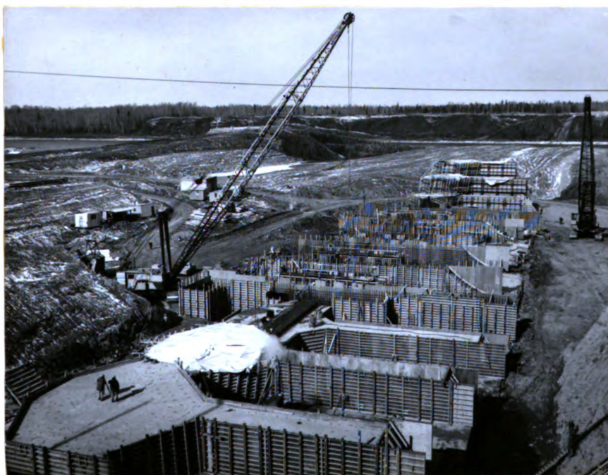
Figure 9. Buttress and spillway structures of the dam looking west.
