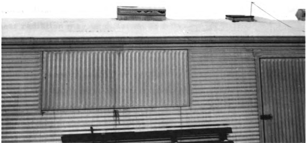
Figure 15. Snow melted on the roof where the warm room air escapes to the attic. Moisture trapped in the ridge vent. The feed is supplied to the feeder through the shutter to the right. M.S.U. Photo No. 63188-9.
