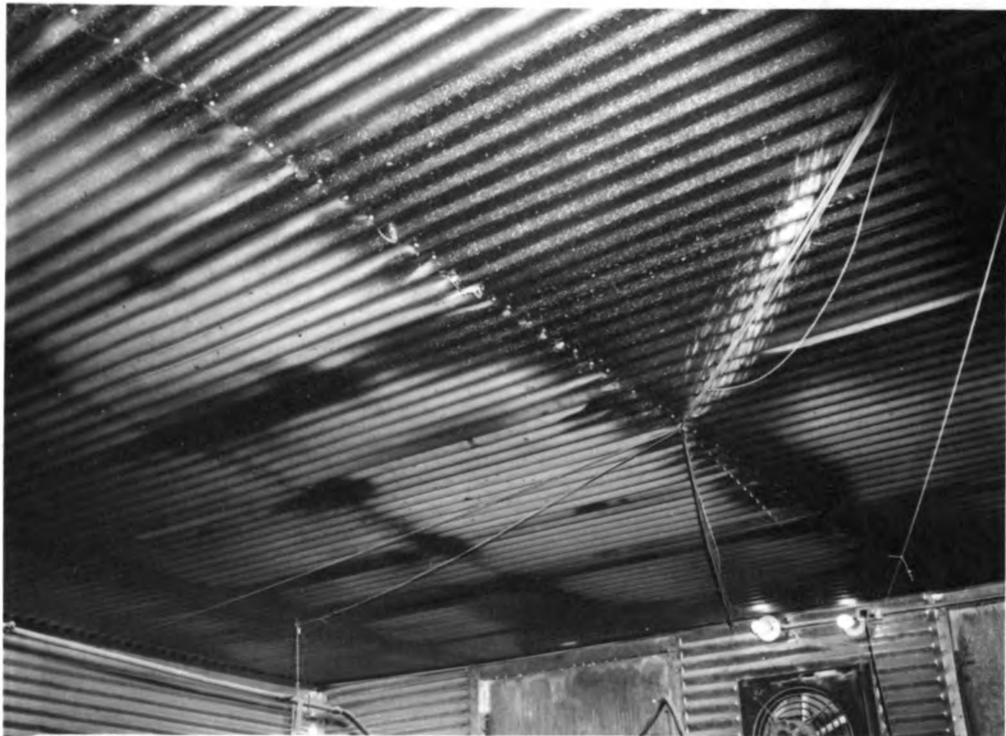
Figure 17. Condensapattern detect deficiency in thermal insulation. M.S.U. Photo No. 63188-2.
