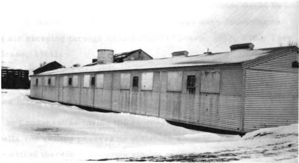
Figure 14. The hog house seen from the lagoon side. The ice covered the lagoon close to the building till the general icemelting in the area. In mild weather a clearing of up to 1 in. appeared between the building and the icecover on the lagoon. M.S.U. Photo No. 63188-5.
