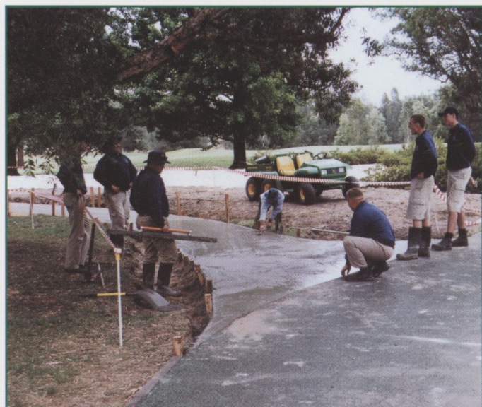
Staff finishing concrete path
