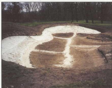
A completed bunker prior to sodding
