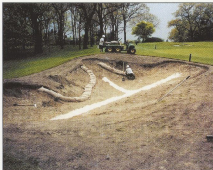
Placing the burlap bags around a fairway bunker
