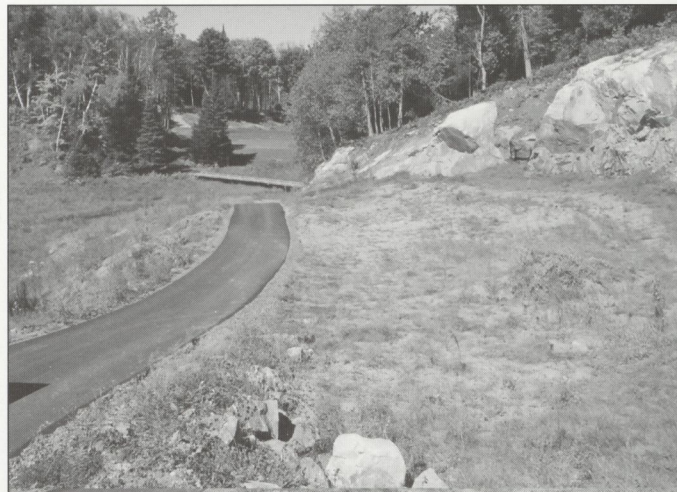
New asphalt cart path through former 15th green site
