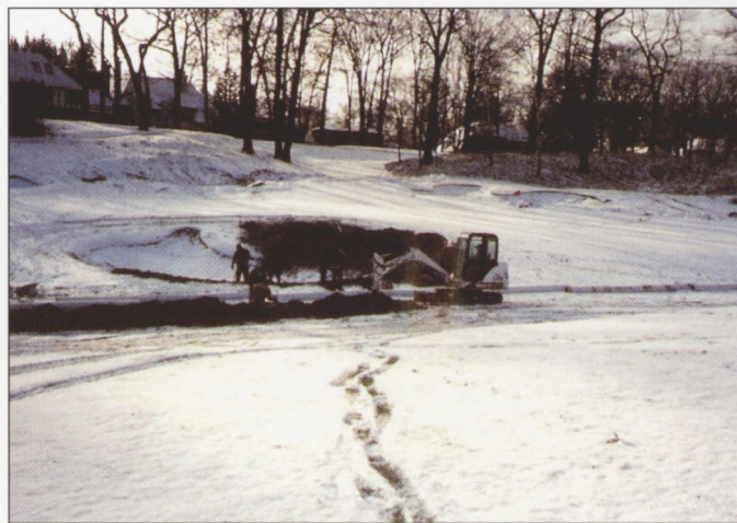
Installation of the drain in front of the third green.
