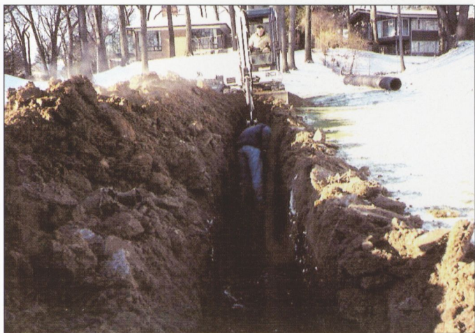
Installation of the drain in the tenth fairway.
