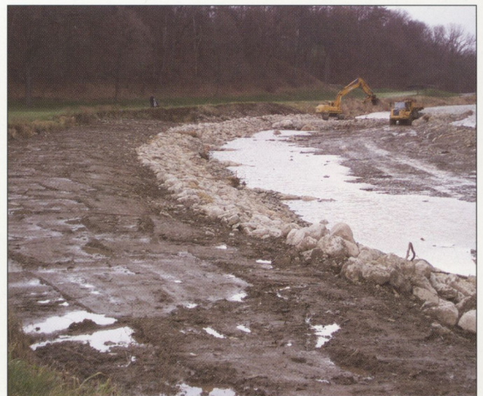
Construction of new bank beside ninth hole
