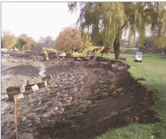
Construction of new bank beside fourth hole
