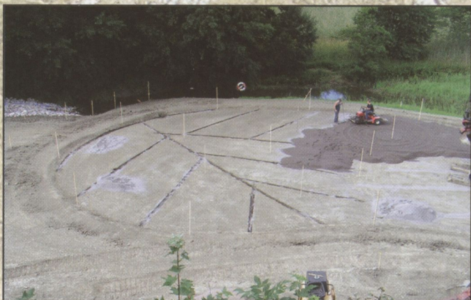
Typical herringbone drainage system and gravel layer on USGA green
