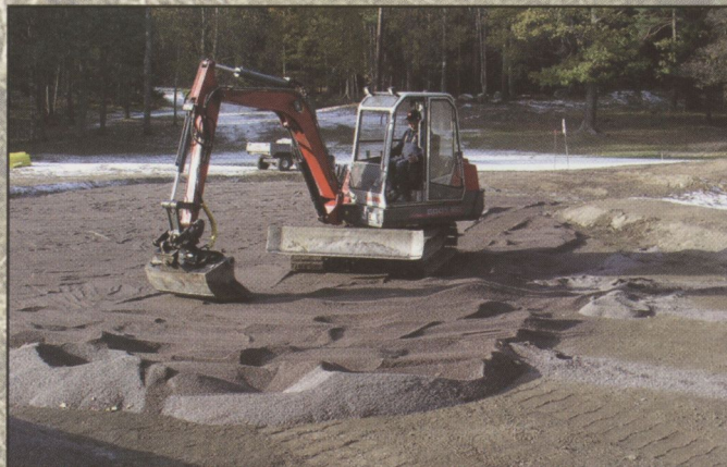
Spreading gravel layer with excavator
