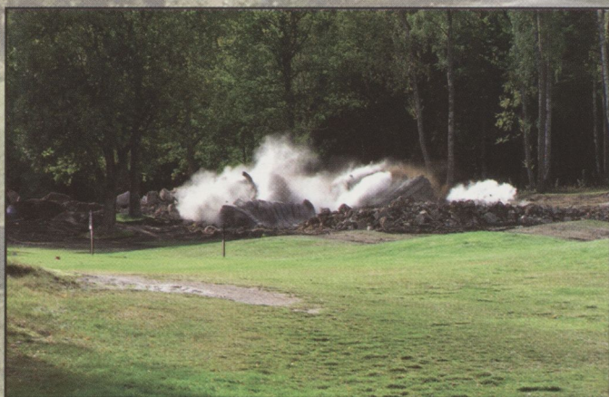
Blasting bedrock to prepare green site for shaping
