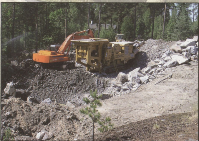
Crushing rock from green site after blasting for use on transportation roads
