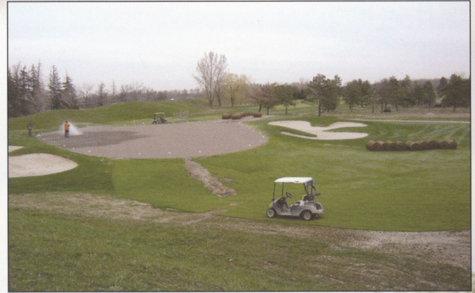
Prepping 6 th for sod
