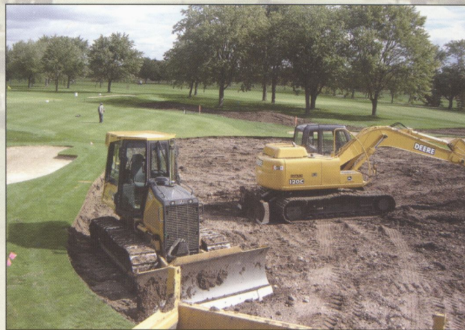
Excavation on 11 th
