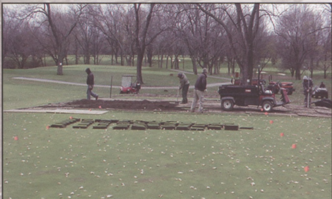
Existing greens drainage in progress.
