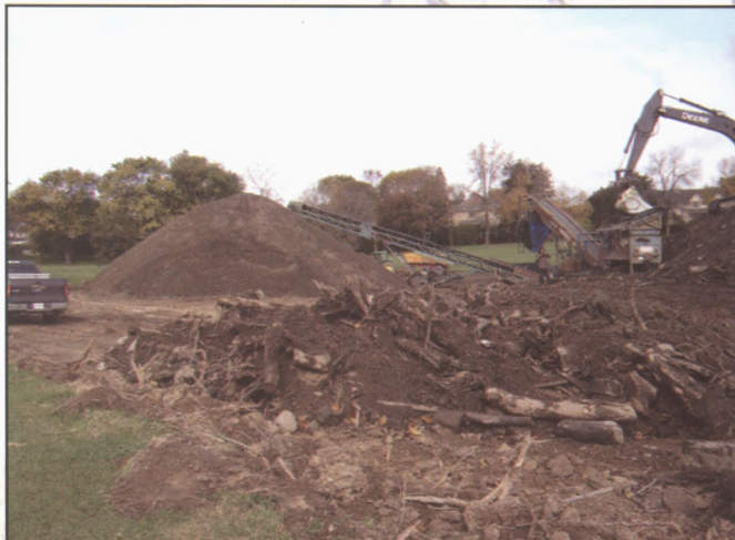
Sorting through the organic matter in the proposed reservoir area between holes 12 and 13
