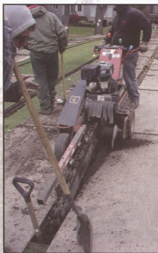
Picture on left - Existing greens drainage in progress.
