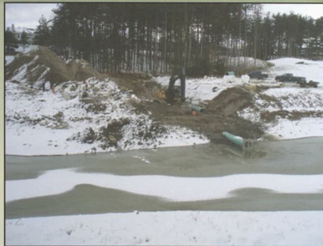
Intake in irrigation pond leading to wet well
