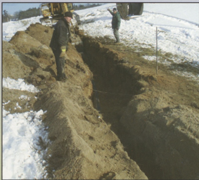
Trench cave in during well transfer line install.
