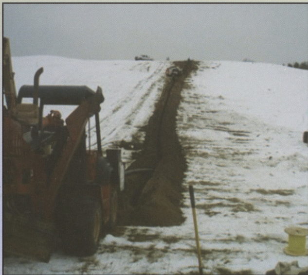
Well transfer line being trenched in.
