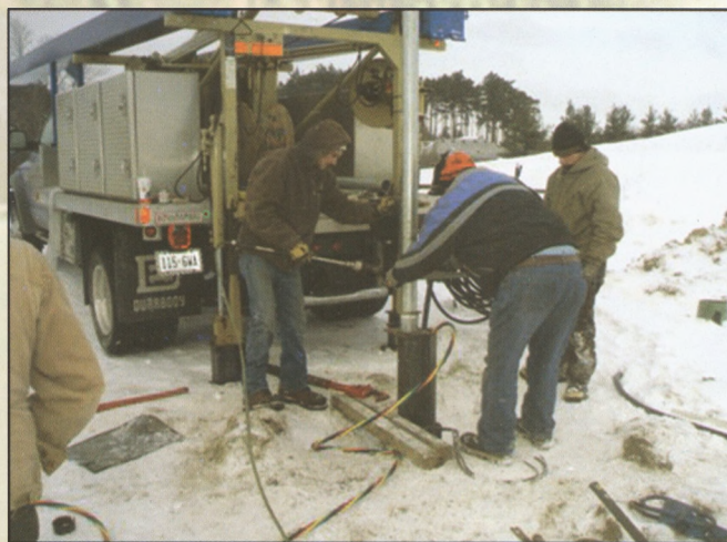
New 25 hp pump being installed
