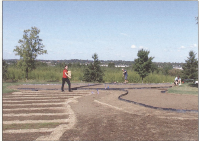
Planting the putting green. Note the temporary plastic edging used to separate the grass species.
