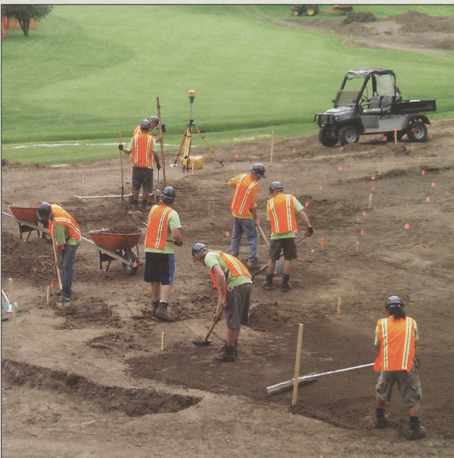
Staff are matching the final grade of the new 11th green to the same grade as the original green.
