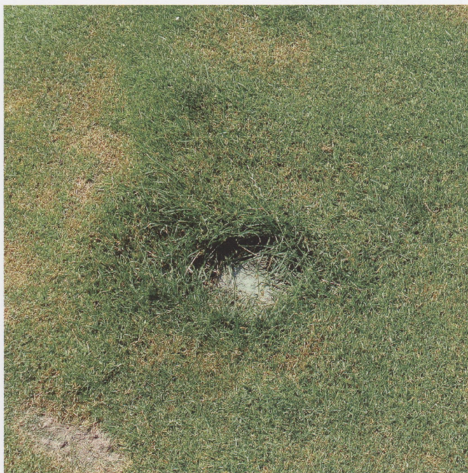
L-R: Ring around a head showing uneven water distribution due to aging equipment. Head sitting lower than it should a few months after repairing an irrigation break, resulting in poor distribution and water pooling in the low settled area.
